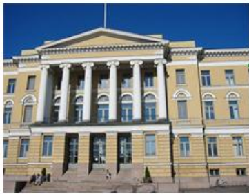
Main Building (front view)
