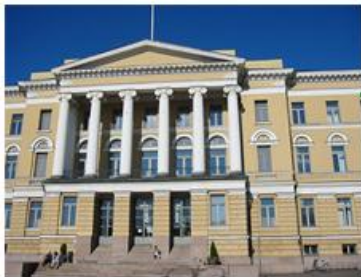
Main Building (front view)
